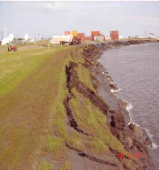
Kwigillingok: Erosion along barge landing site on Kuskokwim Bay in 2011. Yellow plastic poles are placed along the bank to measure rates of erosion.
